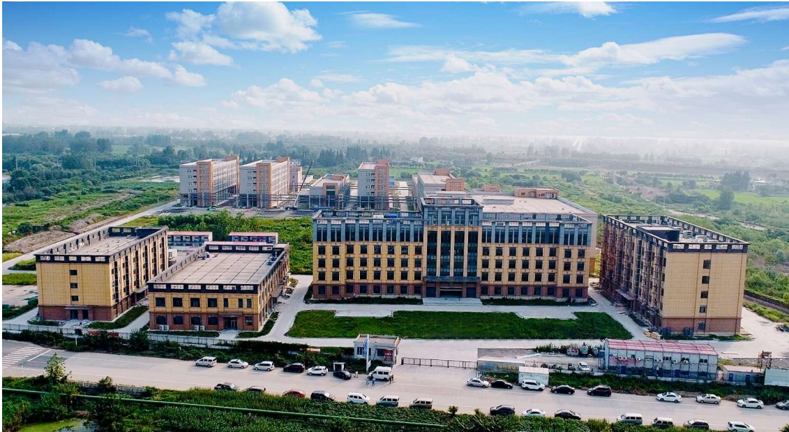
Front view of Yangzhou Aurisco Pharmaceutical Co. Ltd
